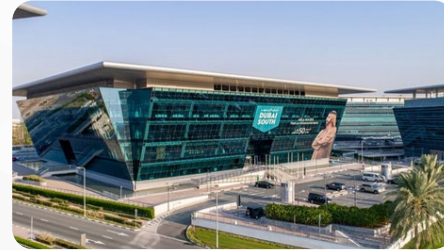
DWC Headquarter Building, Dubai, UAE
