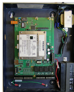
After Installing T-RB-603
