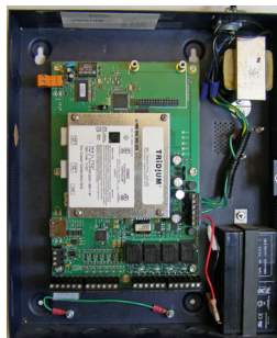
After Installing T-RB-603
